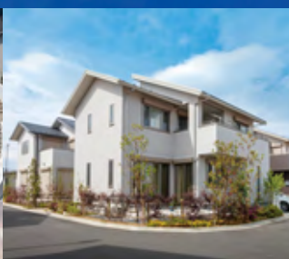
Power lines have been placed underground to enhance aesthetic appearance, earning positive reviews from customers
