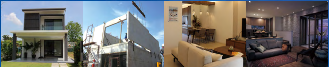
PanaHome's new W-PC construction method, used here in a prototype link house, will facilitate the construction of distinctive houses that feature exceptional heat insulation, ventilation, water resistance and coordinated interior décor
