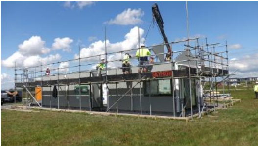
Construction in progress at the site
