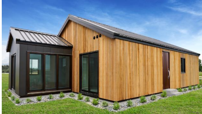
Photo of the prototype standalone house, taken from outside
