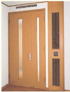
Air cleaning tower (to the right of the door)
