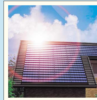
Solar power generation system
