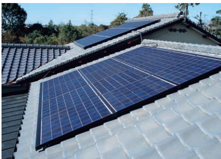
Eco-Life remodeling: solar panels on the roof of a home
