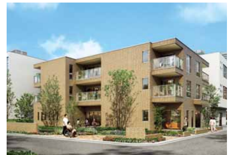
Urban three-story apartment complex for seniors with nursing care services provided
