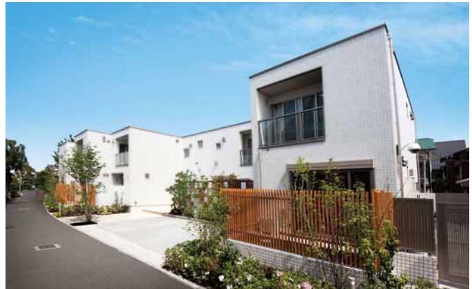
Lacine Inokashira , an urban apartment complex for women with a common ‘community zone’ and enhanced security features
