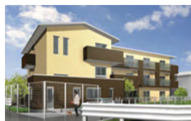
Panasonic Group-operated housing complex for seniors with nursing care services provided
